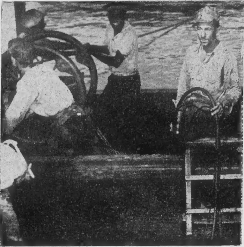
Taking and giving signals through the ropes to a diver under water, Alberto Rincones is traha como yudador di buzo na e reparacionnan na Drydock cu repairs recently completed. Handling an exacting job, he did the work for several months after the regular Crandall Engineering man had in leave because of illness.
